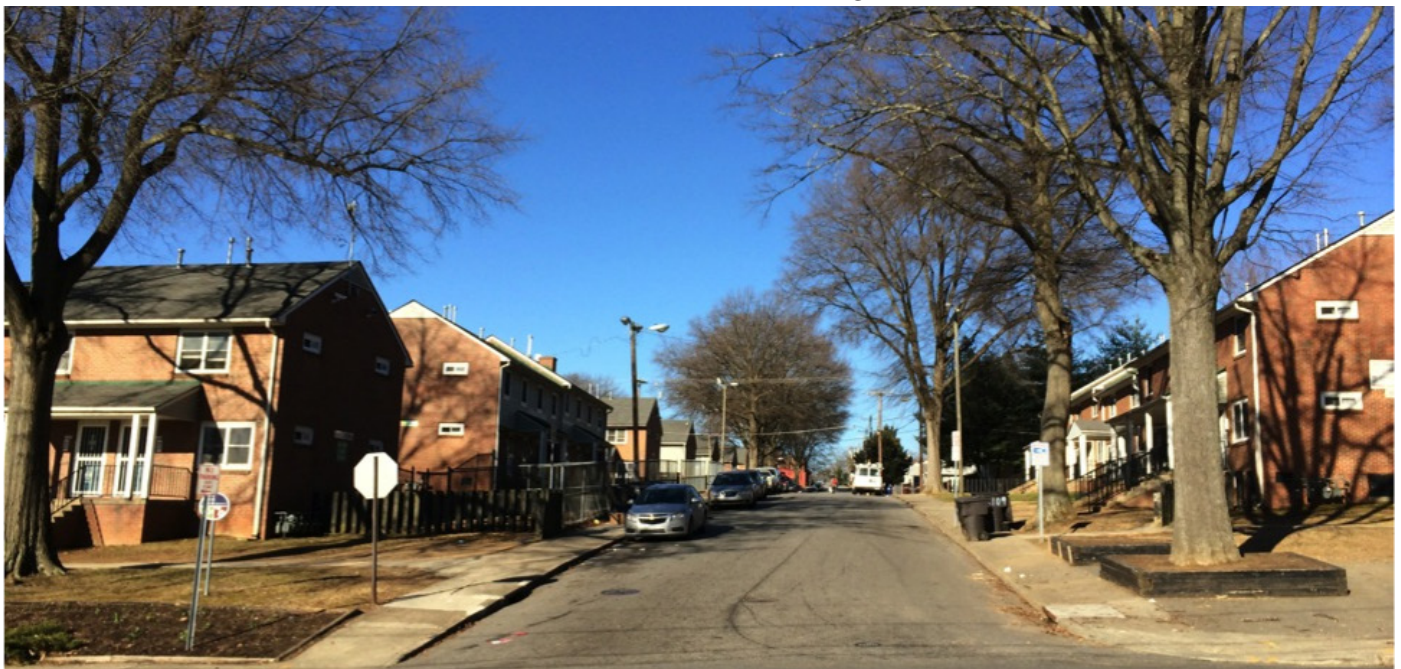
Existing conditions in the Cleveland Avenue Neighborhood
