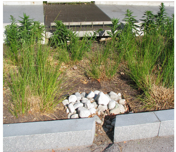
Curb Cuts for Stormwater Capture
